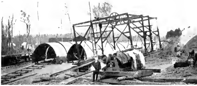
Inside forms and carrier for outside forms.
